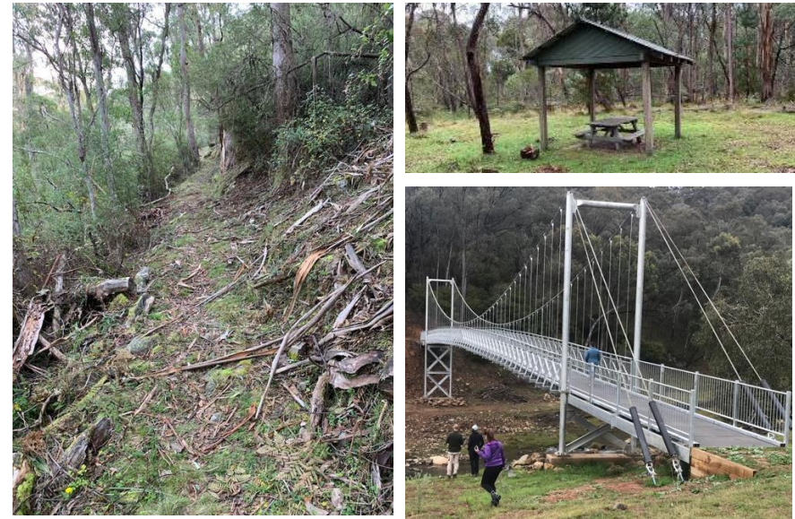
Figure 9.1.1 Examples of track surface, shelter and new Coppabella Creek Bridge
